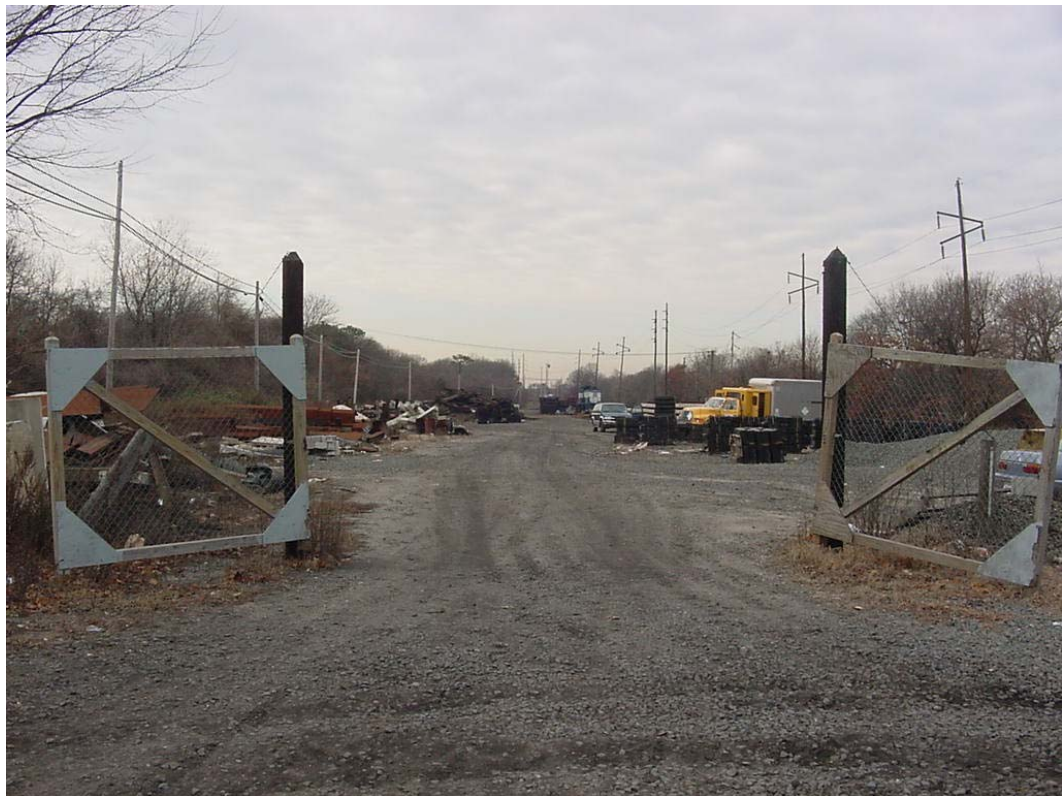
Figure 2: Sayville site—Joint MOW/freight use. Not large enough for yard.
