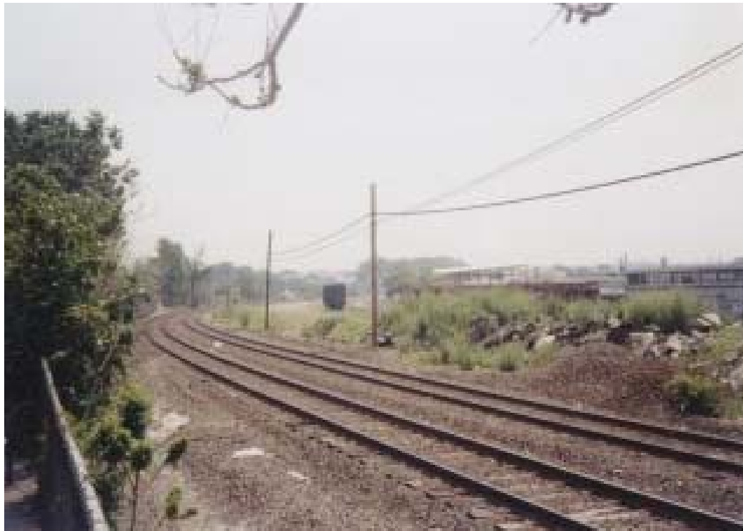
Figure 16: Maspeth site (east view)—low rail freight use. Possible expansion for rail freight.
