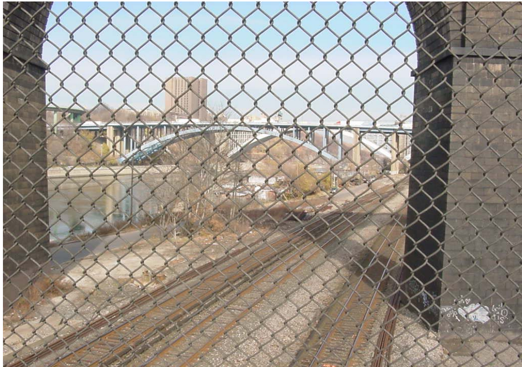
Figure 10: Highbridge site—Occupied. Possible transload.
