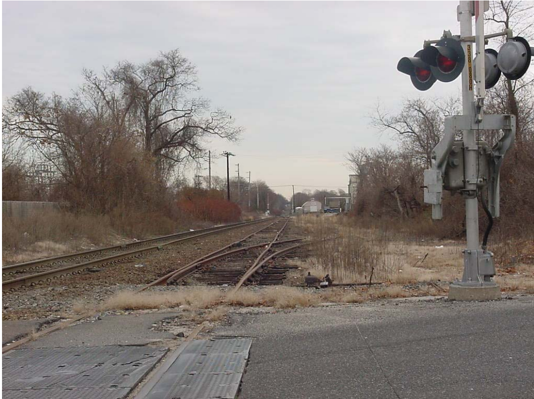
Figure 4: Eastport site—Currently used for freight. Not large enough for yard LIRR maintenance-of-way forces utilize the site periodically.
