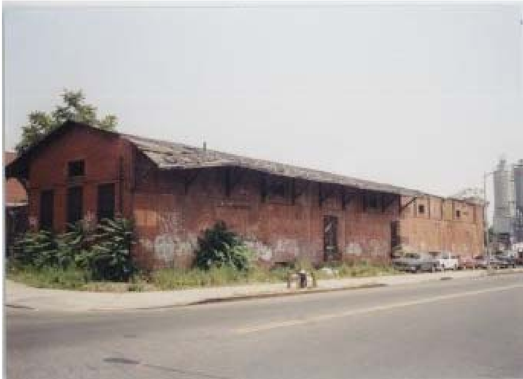
Figure 6: Bushwick site—Hemmed-in by industrial buildings. Not useful for yard.
